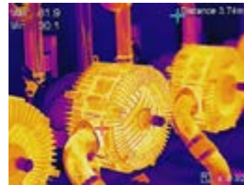
Mechanical Equipment Inspections
